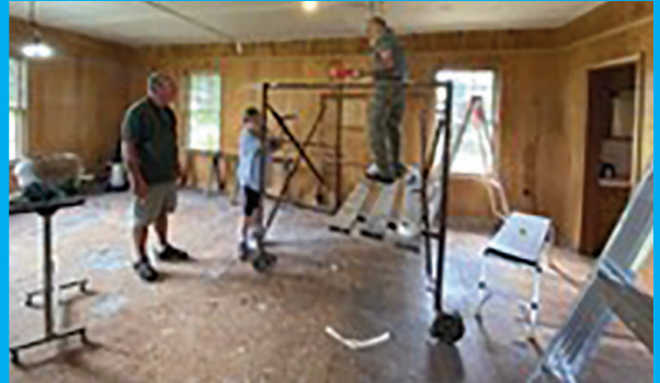
Random pictures of the work in the Home Theater Room
